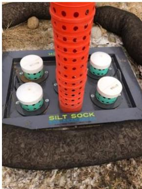
In two other blind inlets, there are existing Hickenbottoms, each of which has been fitted with a Silt Sock wood chip ring protecting an inner ring filled with MetaMateria.
